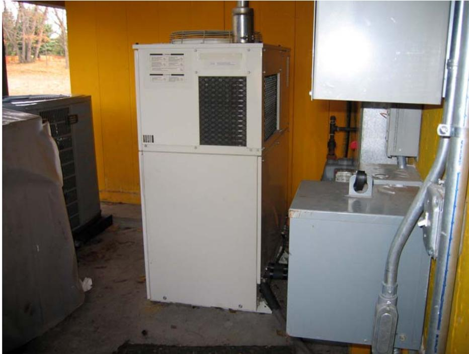
**Figure 1-1. Current Installation of Aisin Seiki G60 Cogeneration Unit at Hooligans**
