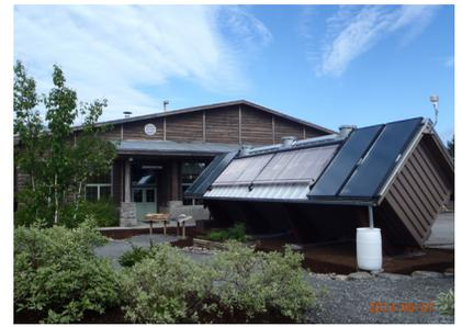
The pellet storage bin is a re-purposed shipping container that also supports a solar thermal hot water system. Credit: NYSEDA.
