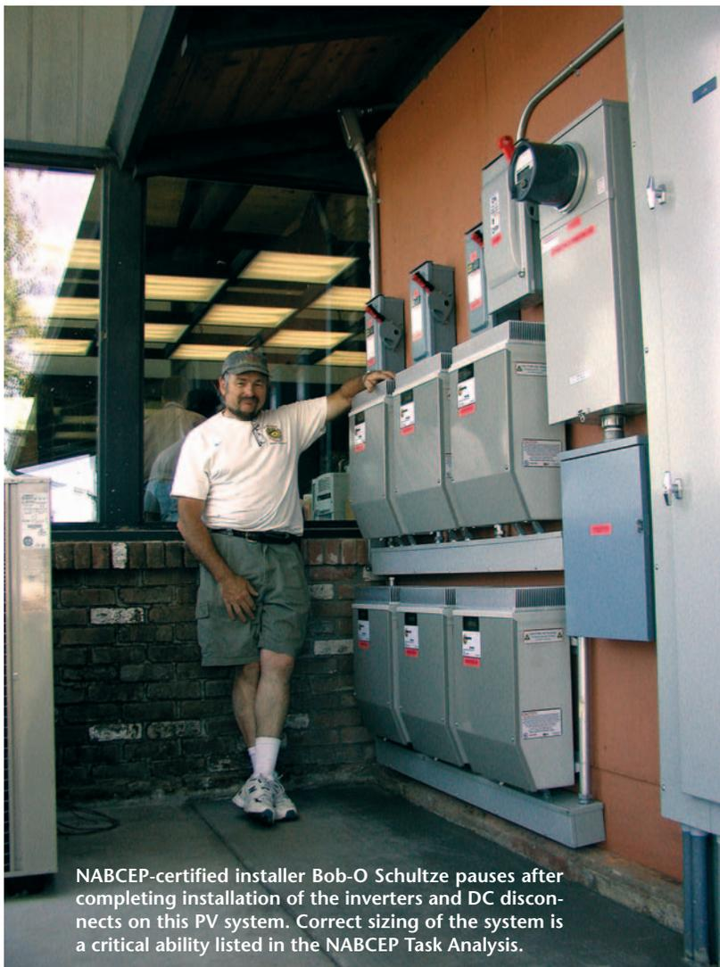
NABCEP-certified installer Bob-O Schultze pauses after completing installation of the inverters and DC disconnects on this PV system. Correct sizing of the system is a critical ability listed in the NABCEP Task Analysis.
