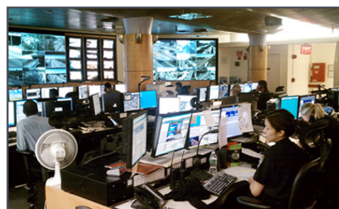
KLD's Advanced Control Decision Support System communicates traffic conditions in real time to operators at traffic management centers such as this one, at NYCDOT, where they can then make adjustments to signal timing in a given area.
