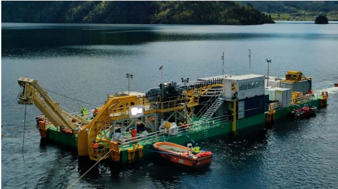
Figure 86: CLB in Operation
