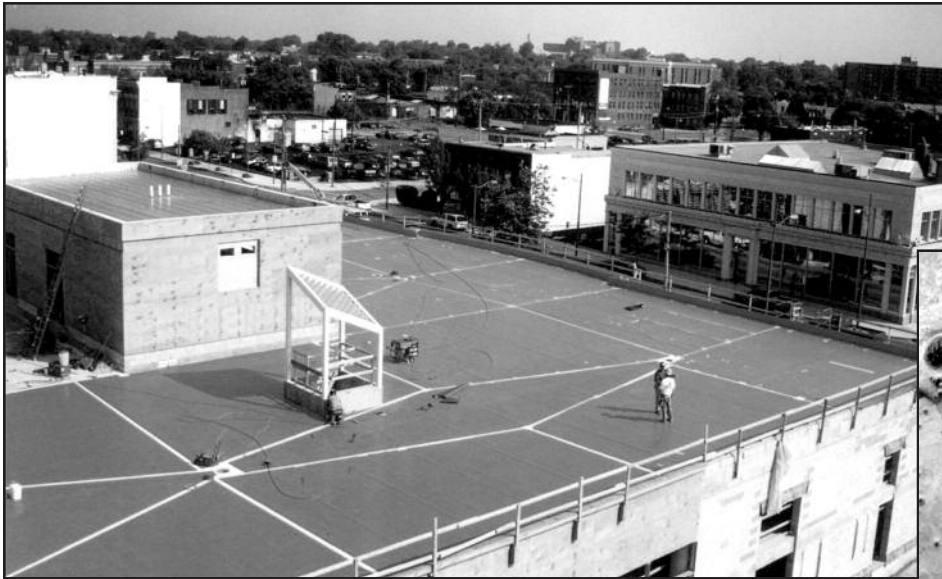
Figure 6 – Compartmentalized installation of single-ply PVC membrane.
