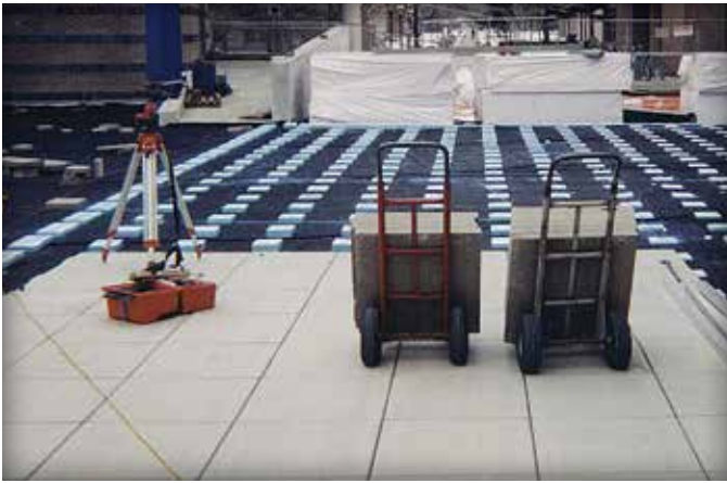
Figure 6. Foam pedestal system
