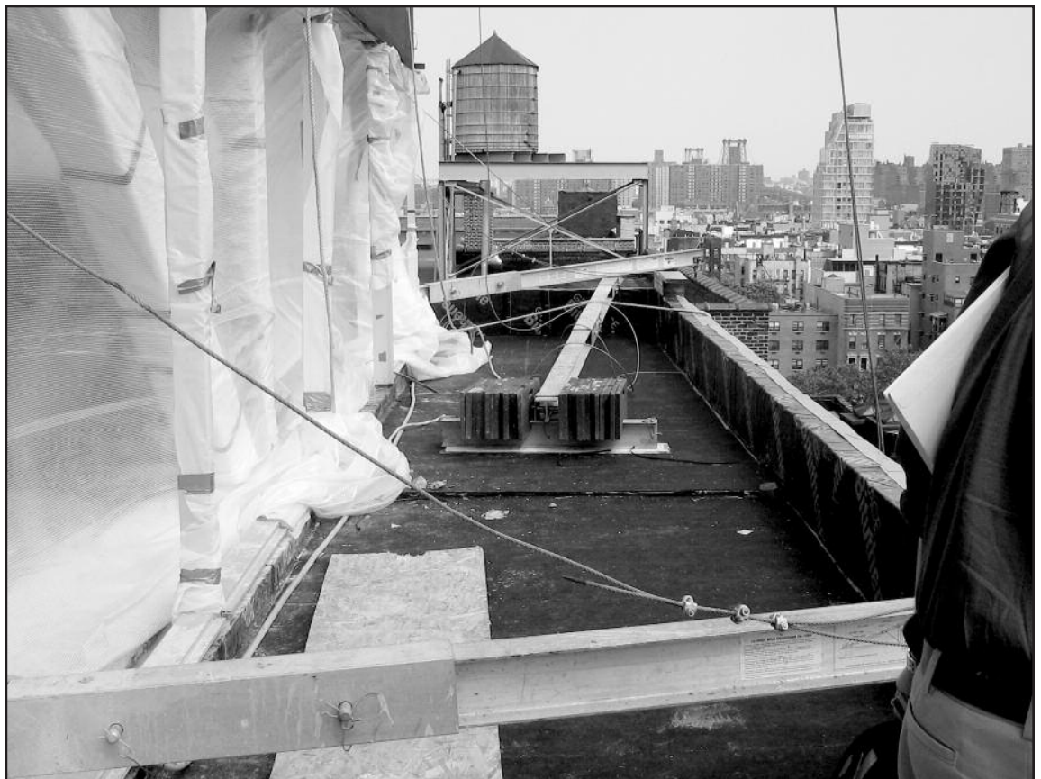
Figure 10 – Construction activities over protection board.
