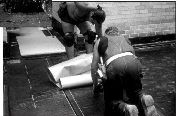
Figure 5 – Application of self-adhering modified bitumen membrane.
