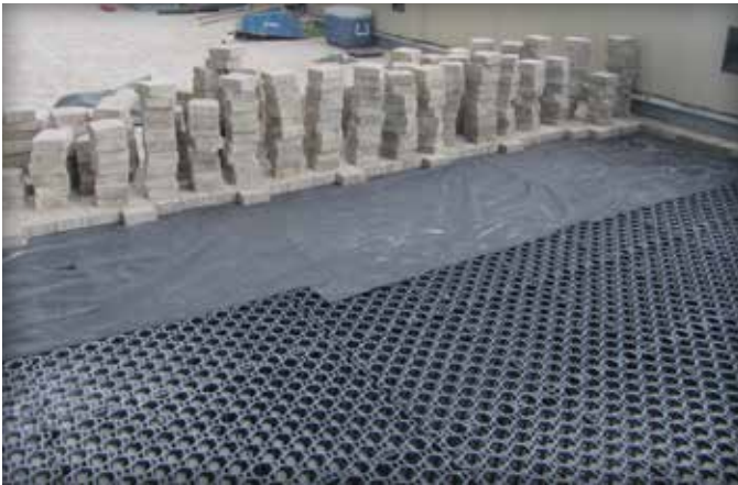
Figure 7. Concrete pavers on geotextile over plastic grids
