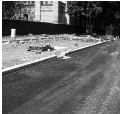
A Asphalt setting bed, ready to receive hexagonal asphalt pavers.
