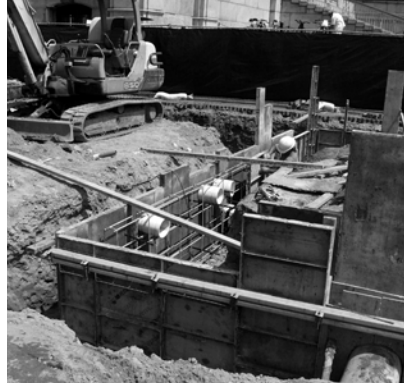
A Construction of concrete retaining walls.
