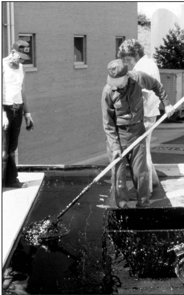
Figure 4 – Application of a coal tar pitch waterproofing membrane.
