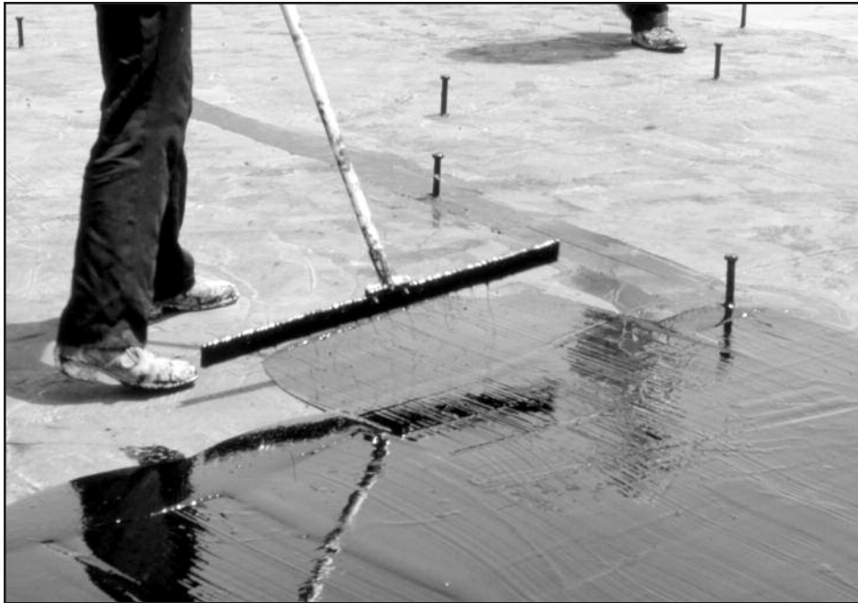
Figure 9 – Squeegee application of cold-applied liquid membrane.
