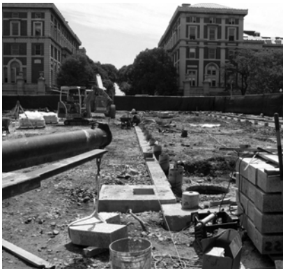
A Installation of granite curbs.
