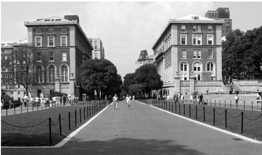
A The reconstructed pedestrian street. The redesigned paving system can withstand frequent, heavy pedestrian traffic, as well as vehicle use, while preserving the aesthetic character of the original plaza.
