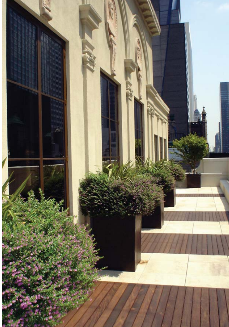
This large penthouse terrace was designed as an outdoor environment to complement a multi-million dollar apartment high atop the New York City skyline, with multiple levels requiring exceptional waterproofing, especially around the flashings.
