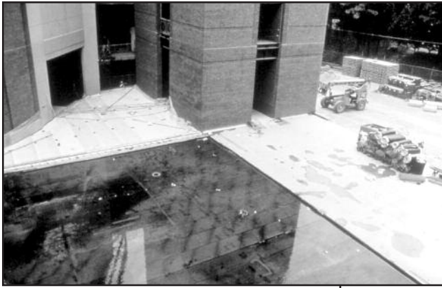
Figures 18A and 18B – Flood testing. (Sketch courtesy of ASTM International.)
