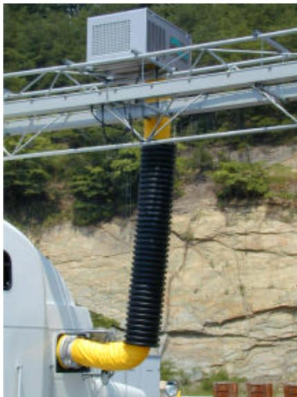
**Figure 3. Truss mounted HVAC system and ducting**
