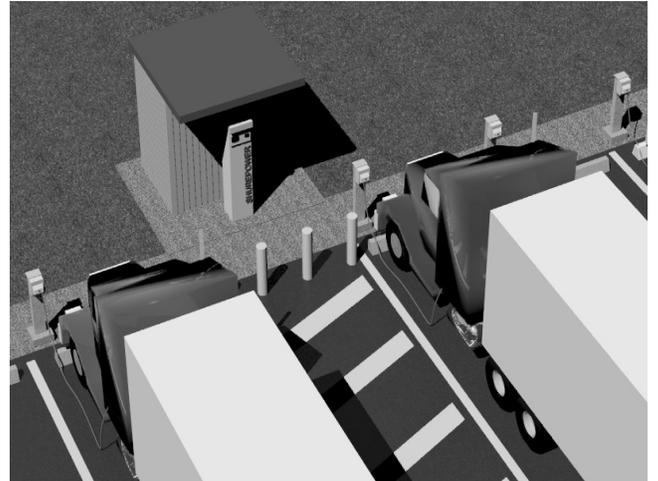
**Figure 2: Shorepower control kiosk and control building**
