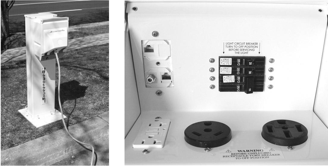
**Figure 3: Shorepower pedestal with electrical, cable TV, Internet, and phone connections**
