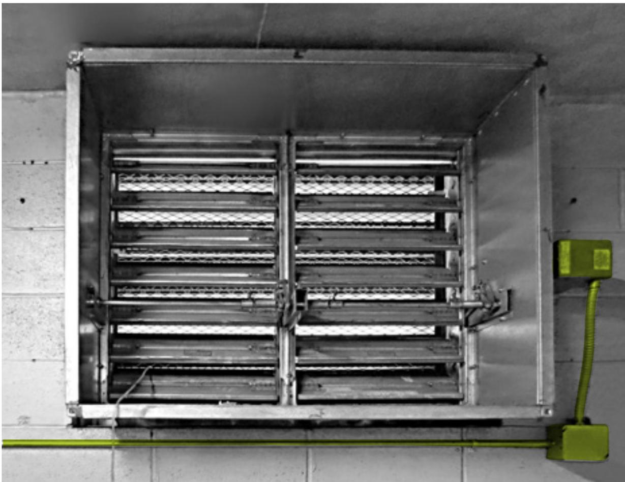
**Figure 4:** A motorized, fully closing vent
