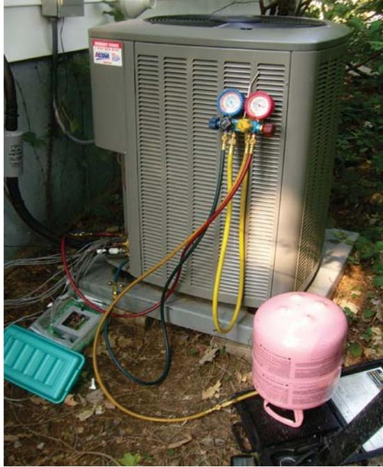
**Figure 3-4 Refrigerant Charging by Gravimetric (Weight) Method.**
