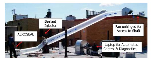
Figure 1. AEROSEAL installation set-up on roof a demonstration building.
