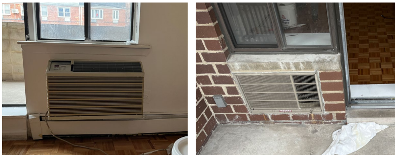
Figure 4. Site 2 Air Conditioner Sleeves
