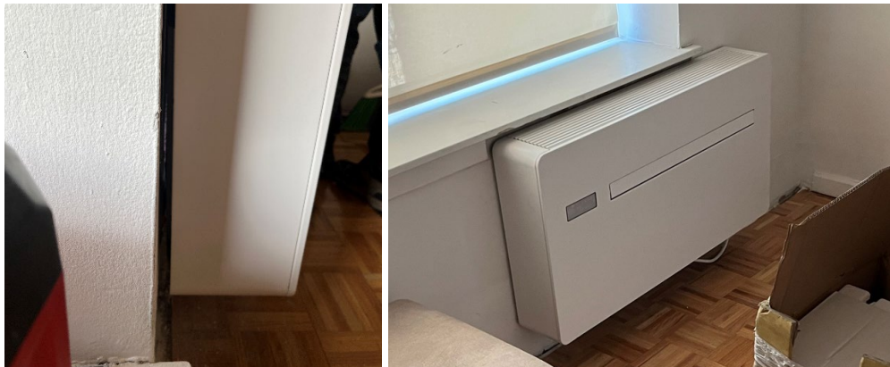
Figure 12. Installed Heat Pump Units
