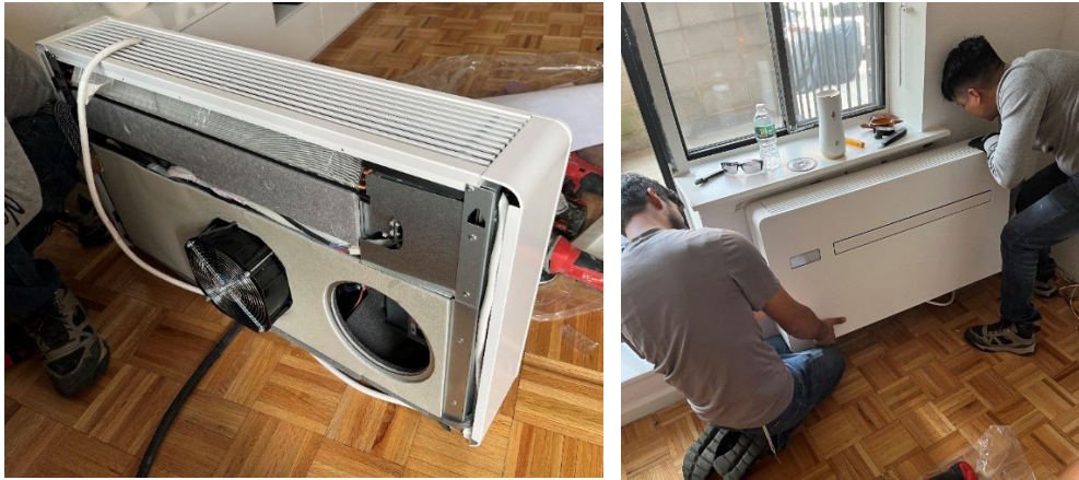
Figure 12. Installed Heat Pump Units
