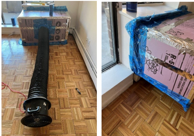
Figure 13. Sleeve Air Leakage Testing
