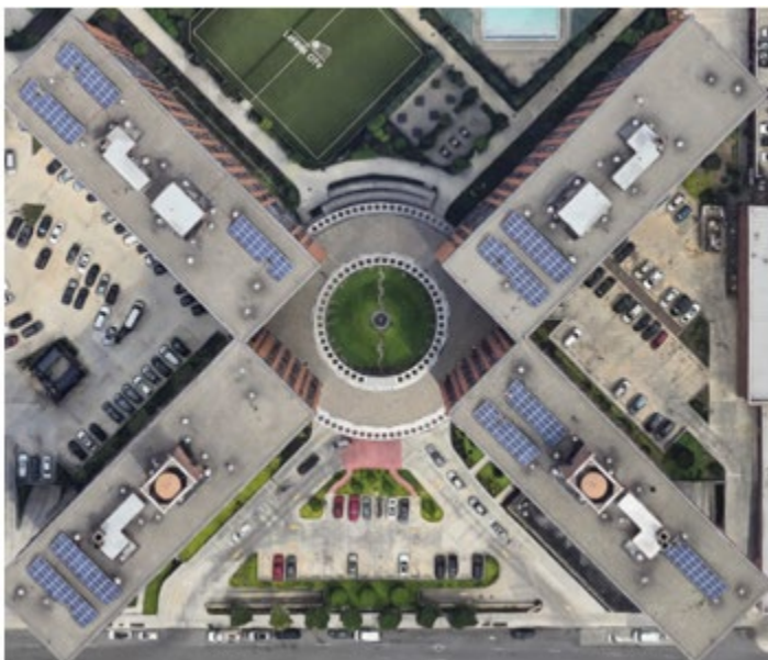
Figure 20. LeFrak City: Building Rooftop Solar Panels
