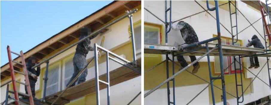
An additional one-inch thick by four-inch wide layer of EPS is used to form window trim (Figure 7). This was done primarily for aesthetics, but also to help improve R-value in an area where wall cavity insulation is compromised by additional framing. Other applied shapes can be used to create architectural forms as desired.
