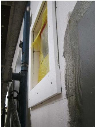
The gray basecoat is troweled on over an embedded layer of reinforcing mesh, which provides a durable surface (Figure 8). Additional layers of mesh can be added to increase impact resistance. The basecoat is applied over the formed window trim and edges of the EPS panels, embedding the yellow mesh around windows and other penetrations (Figure 9).
