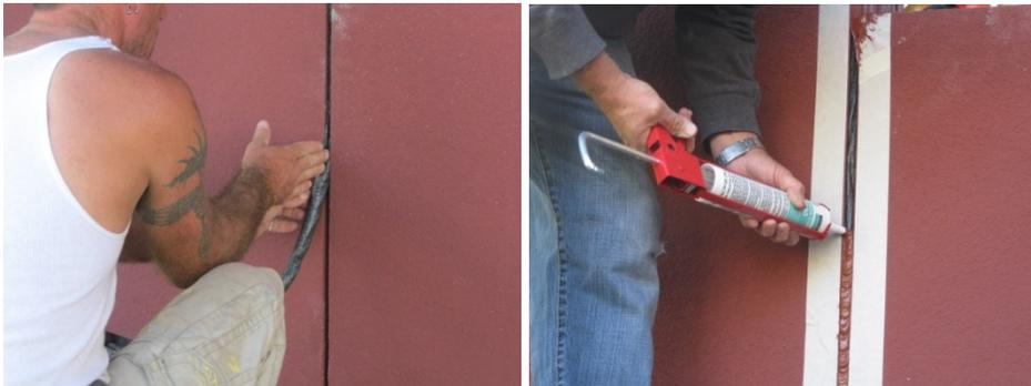
Panels were installed across the entire building, including the solar PV closet and solar thermal tank enclosure to produce a uniform thermal barrier and appearance across the entire building façade (Figures 27, 28, and 29).
