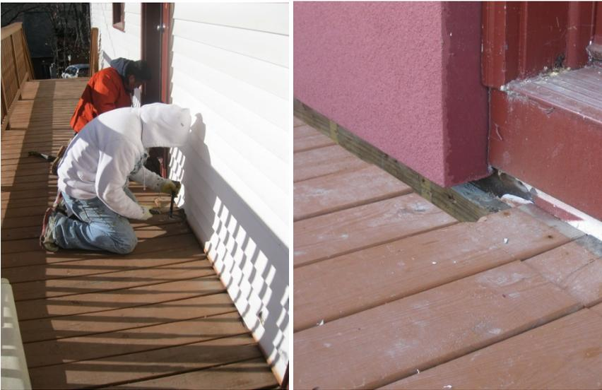
At the first-floor masonry, all brick protrusions were chiseled back, creating a level surface upon which to install the EIFS. Existing vinyl siding and weather-resistive barriers were removed from the second-floor, exposing the exterior sheathing beneath. Prior to the full application of the liquid WRB, a separate coating, embedded with reinforcing mesh, was brushed into the sheathing joints, as was done at Central Islip (Figure 18).
