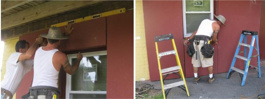
Installation of the foam backer rods ensures a continuous thermal barrier by sealing gaps between the panels. Masking tape was applied to the panels prior to caulking to avoid damaging the aesthetics of the panels (Figure 26).
