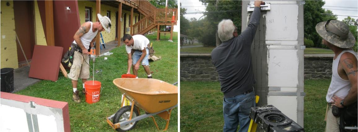
**Figure 23. The lightweight panels are lifted into place by hand and pressed to the wall**
