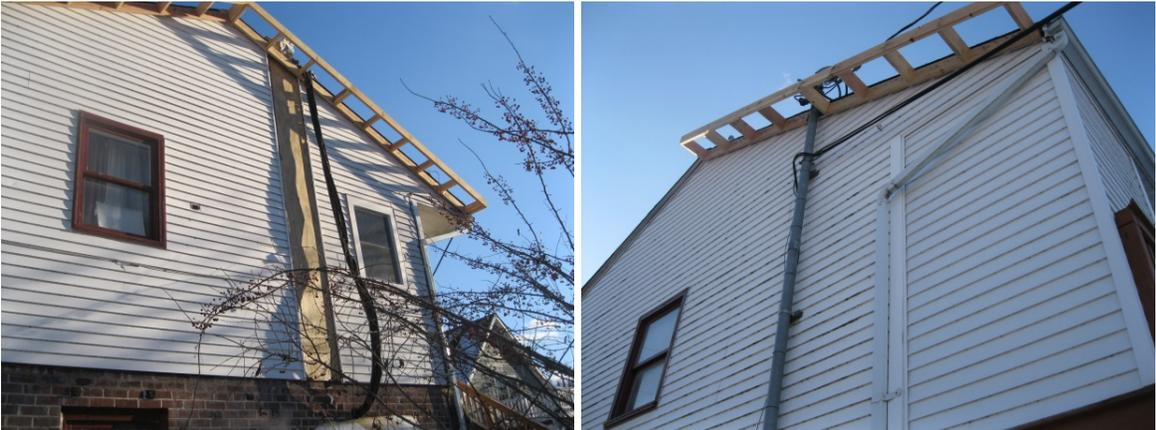
The second-floor walkway deck planks were trimmed back. If left in place, the deck planks would have resulted a thermal bridge along the length of the building between the two floors. By trimming the planks back, the EIFS ran continuously behind the deck, resulting in an uninterrupted thermal barrier. The deck joist against the building was moved out approximately four inches so that the panels could fit behind and remain flush at joints and seams (Figure 17).
