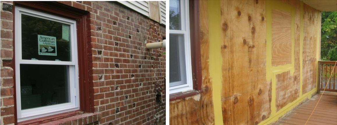
A liquid water-resistive coating was applied to the entire building to prevent moisture from soaking through the brick and entering the interior wall assembly. Once the coating dried, gaps in the brickwork from the chipping of protrusions were filled with spray foam (Figure 19).
