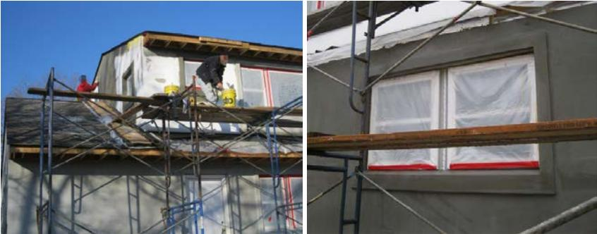
The final step is to apply the finish coat, which includes the color and texture. The material arrives in pails and is first mixed and then troweled on (Figure 10). The final product is shown in Figure 11.
