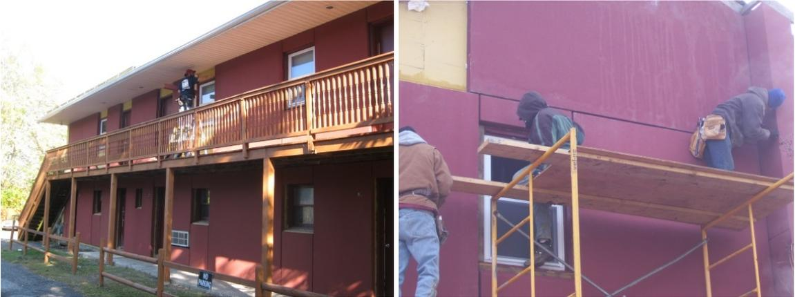
**Figure 28. Following installation of the panels, the roof extension is shingled and finished**
