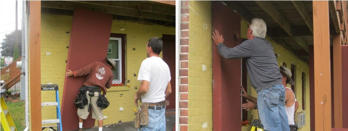
Each panel was prefabricated with metal tabs that can be modified to extend approximately three-quarters of an inch from the edge of the panel and screwed in place. This allows for provisional panel support during the adhesive curing period (Figures 24 and 25).
