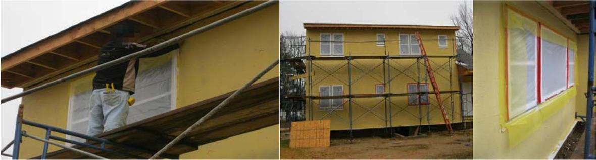
Sections of EPS insulation, 4-inches thick and measuring 2×4 ft, are adhered to the walls. Where necessary, the backside of the panels are rasped to conform to irregularities in the substrate wall. The EPS joints are smoothed out (Figure 6). Smoothing the joints between EPS foam panels is essential for getting an even finish coat that avoids telegraphing joint lines.
