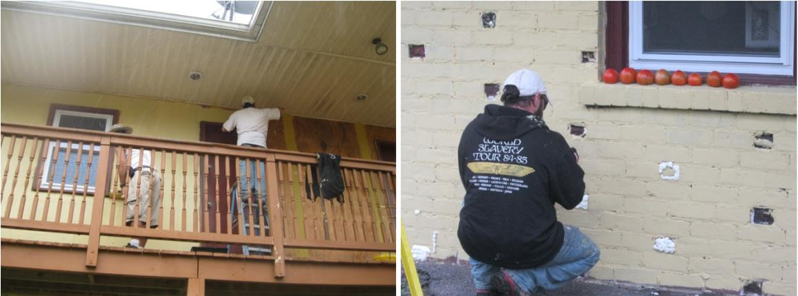
The nature of the retrofit process necessitated on-site modification of the panels at uneven or protruding portions of the building facade, such as window sills. This was necessary to allow electrical wiring to run through the panels at existing light fixture locations. Therefore, the panels and façade were carefully measured prior to application (Figures 20 and 21).
