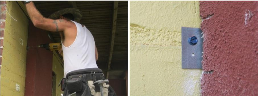
**Figure 25. As panels are applied, they are scrutinized to ensure a close, level fit**
