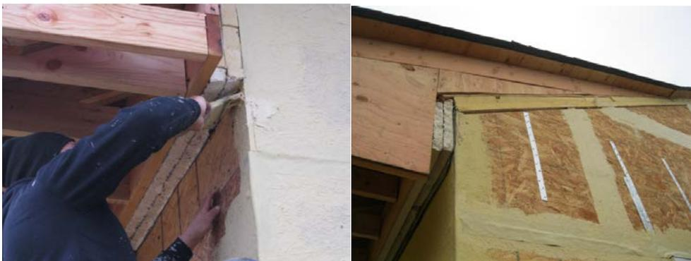
An approximately 12-inch wide strip of reinforcing mesh is left hanging at all four sides of the window openings (Figure 5). It will later be wrapped around the edges of the EPS panels, protecting them at all exposed edges. This obviates the need, in standard installations, for any additional window trim to be built out to the thickness of the added EIFS, thus eliminating a step required for other wall insulation retrofit techniques that use built-up insulation and siding.
