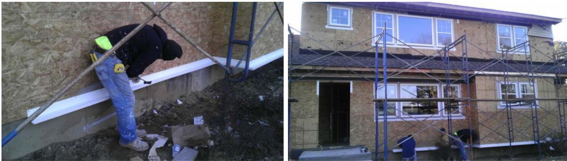
Next, a liquid water resistive barrier (WRB) is brushed onto the sheathing; a layer of reinforcing mesh is embedded into the coating at the sheathing joints (Figure 4). Overhangs at eaves were removed and added back on over rigid insulation to match the 4-inch EIFS thickness. At the gable ends, the roof deck was extended where necessary to match the 4-inch EIFS depth. A metal drip edge was added to direct water away from the rake.
