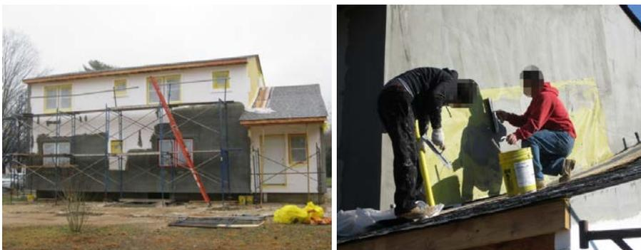
**Figure 9. Basecoat is applied over window trim and edges panels**
