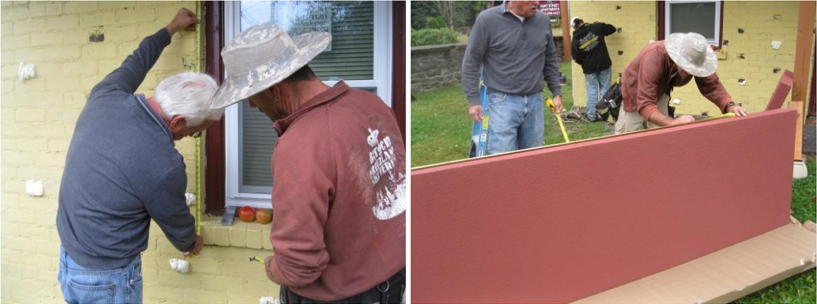
**Figure 21. Notches are cut with a circular saw and adapted to fit protrusions using a boxcutter**
