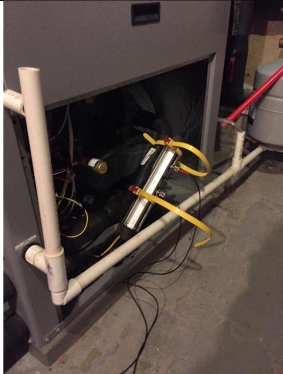
Fuji ultrasonic flow meter installed on 1 inch copper line:
