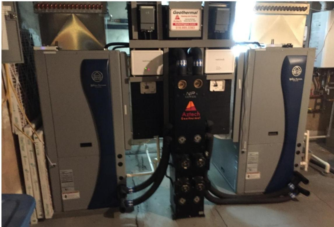
Figure B-1. Two Heat Pumps installed at Niskayuna
