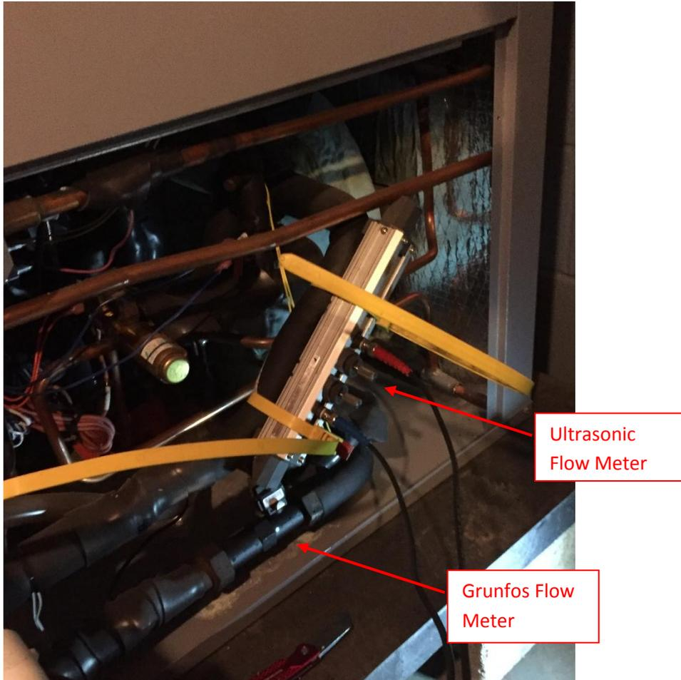
Fuji ultrasonic flow meter installed on 1 inch copper line: Diameter 1.125 in, wall 0.05 in, Copper type L (or 1-1/8 inch ACR) Head spacing: 0.306 in
