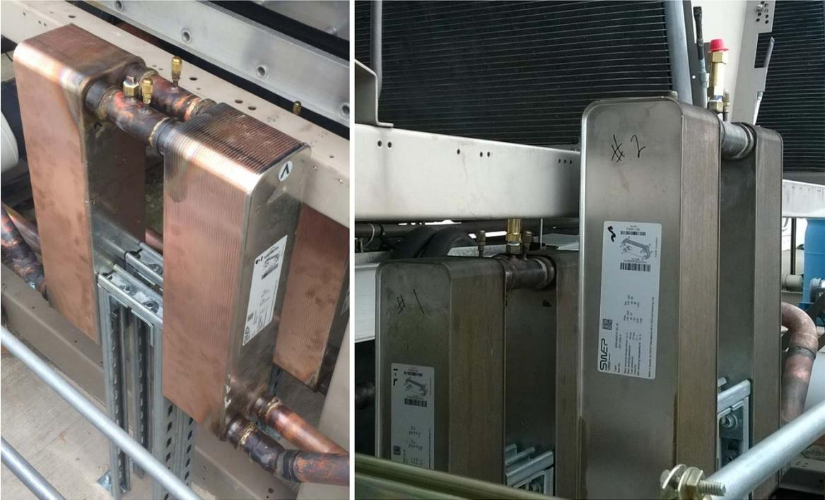
**Figure 6. Subcooler pipes**
