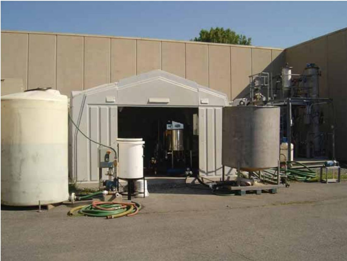
Every other day, approximately 300 to 400 gallons of high-strength waste was batch processed in the pilot DAF unit shown in Figure 2-3. A three-foot diameter, pilot-scale Krofta Technologies Supracell DAF unit was used. A schematic of the system is shown in Figure 2-4. Ashland Drewfloc 2270 was added to the unit at approximately 150 mg/L. The pilot DAF float was pumped to a sludge storage tank, then to the WWTP's existing DAF, and then to the WWTP's existing anaerobic sludge digesters.
