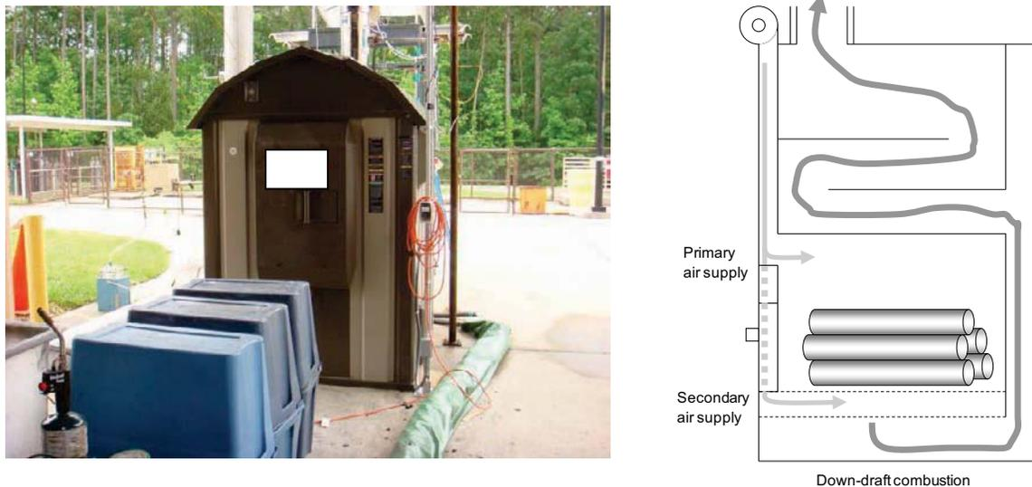
**Figure 2-5. Three Stage HH and Illustration of a Down-draft Combustion Unit.**
