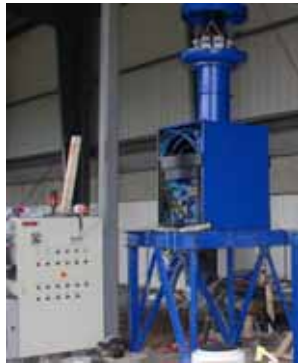
Figure 5. Field Installation of Pilot Squeeze Tower Press
