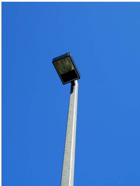
Figure 1-5. Example of a shoebox-style street light
