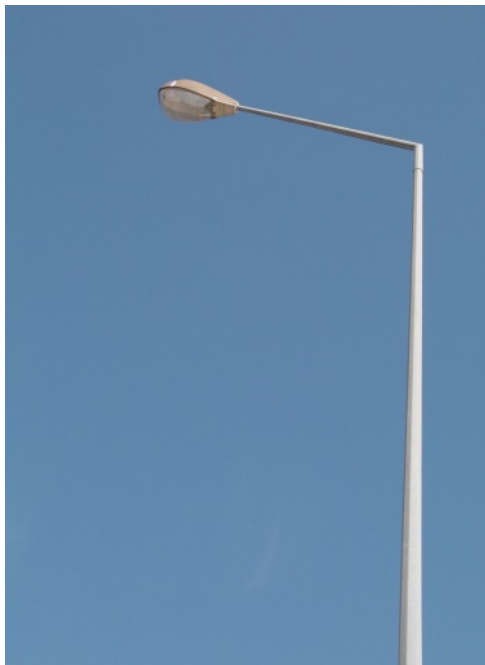
Figure 1-4. Example of a cobrahead-style street light
