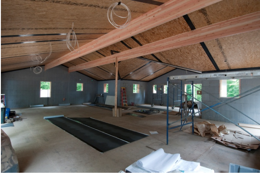
Figure 4. Kraft Home SIPs Installation Complete
