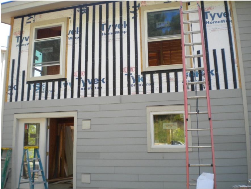
Figure 25. INHS-Ithaca B Vented Siding
