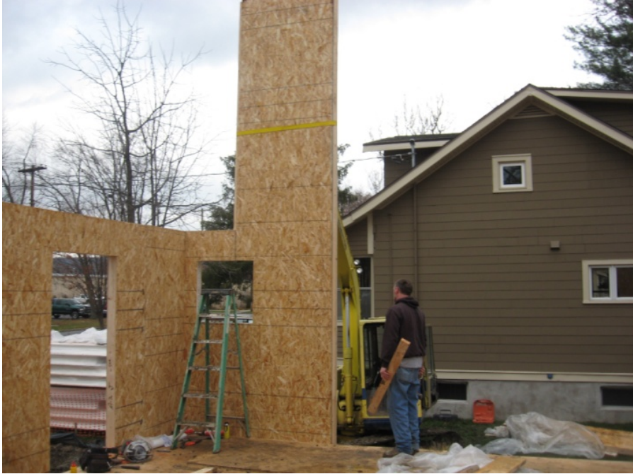
Figure 9. INHS Ithaca A SIPs Installation
