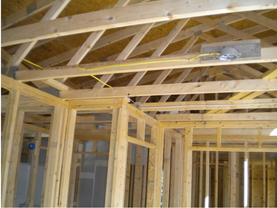
Figure 20. INHS-Ithaca B Trusses
