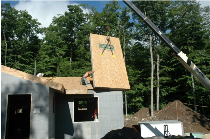
Figure 3. Kraft SIPs Roof Installation
