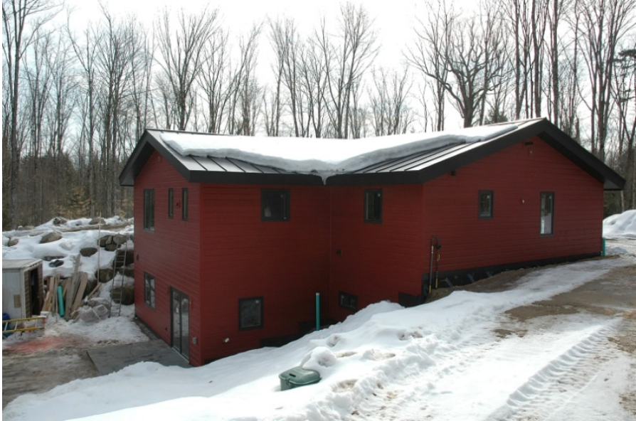
Figure 6. Kraft Home Rear Elevation
