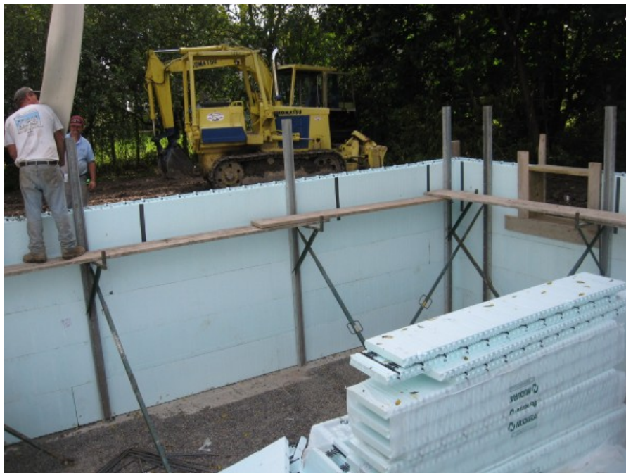
Figure 8. INHS Ithaca A ICF Foundation
