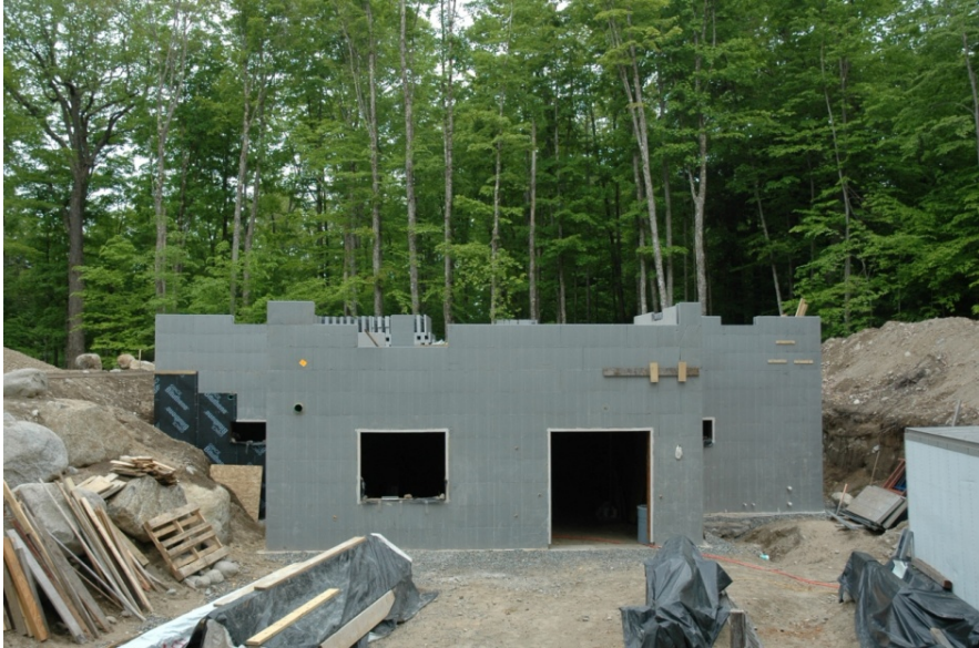
Figure 2. Kraft Neopor ICF Foundation
