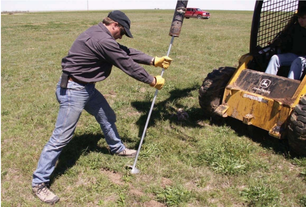
Figure 5-4 Example of an screw-in guy anchor installation. (Source: AWS Truepower)
