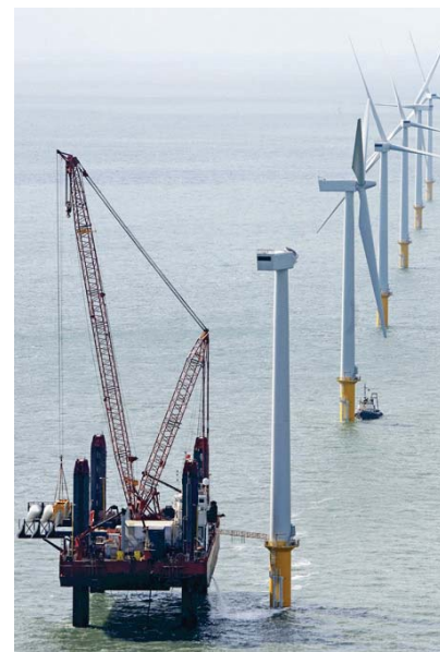
Figure 7.5: Heavy Construction Vessels Installing Wind Turbines 92,93
