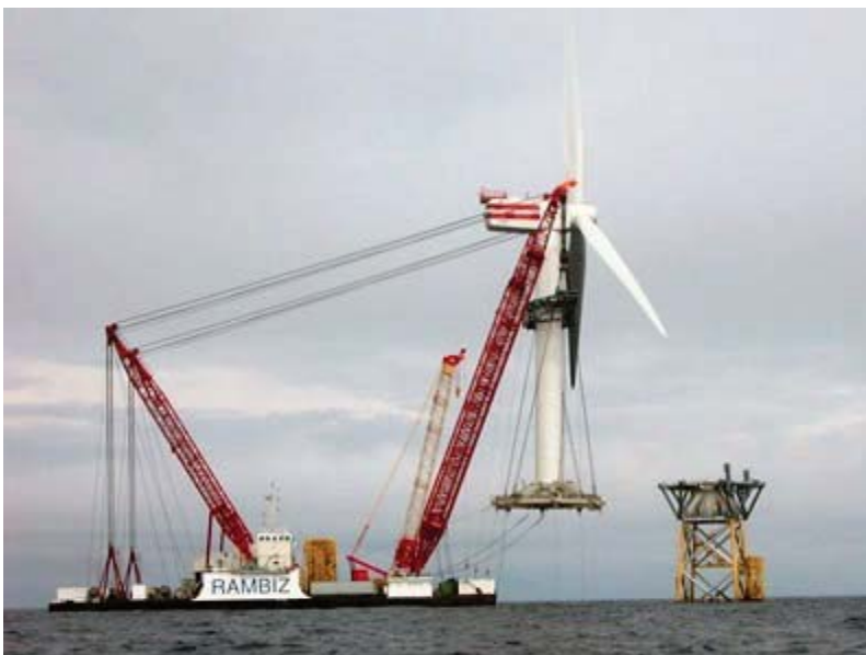
Figure 7.5: Heavy Construction Vessels Installing Wind Turbines 92,93
