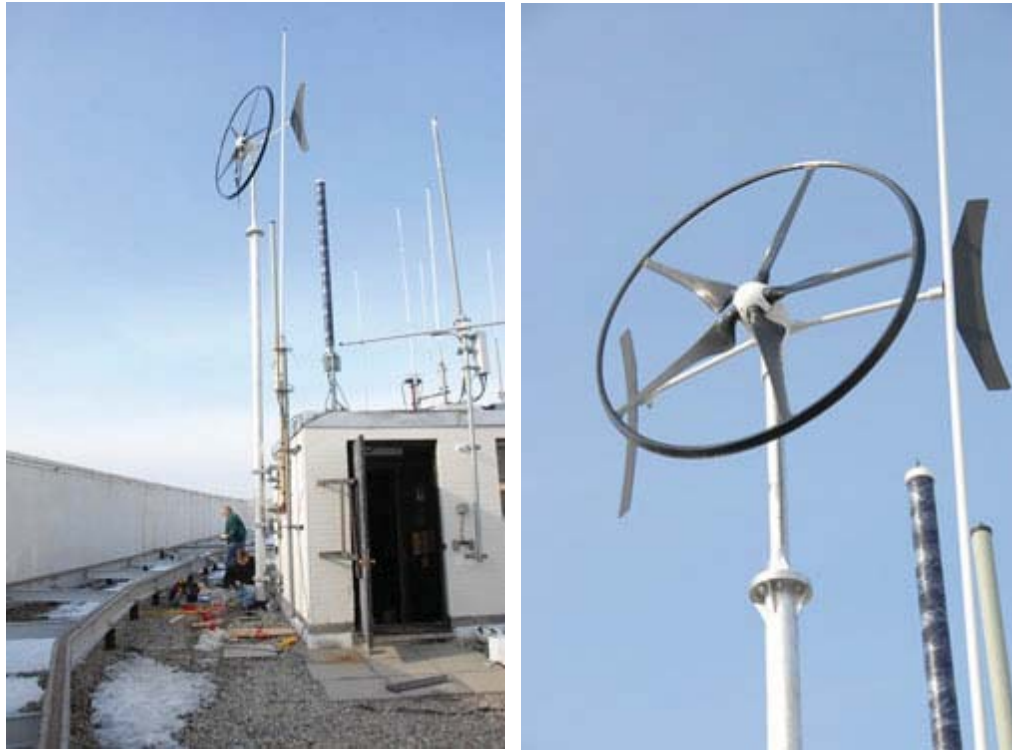
Figure 2.2: SWIFT 1.5 kW Turbine's Mounted on 6.6 m (22 ft) Pole 10
