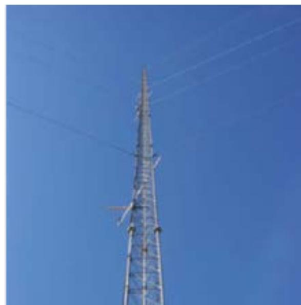
Meteorological masts or towers are typically 60 or 80 meters tall and have monitoring equipment at multiple heights. These towers use anemometers, wind vanes, and temperature sensors to measure the wind speed, wind direction, and temperature. This wind resource data is collected and stored by a data logger for later analysis.
