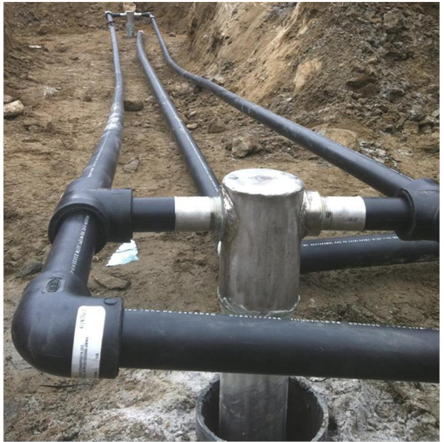
The coaxial fusion head separates flow channels and is connected with the other HPGX loops via standard reverse-return.
