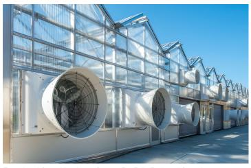
Tunnel and Cross Ventilation System For Fully Enclosed Greenhouses
