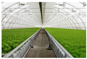
between the poly layers can result in other problems like material deterioration and mold. By using a poly layer that has an IRAC coated inner layer, the condensation is eliminated, and the thermal radiation losses are reduced by up to 20%. The cost difference for an IRAC film-coated poly covering over a standard covering is about \$0.02 per square foot.
