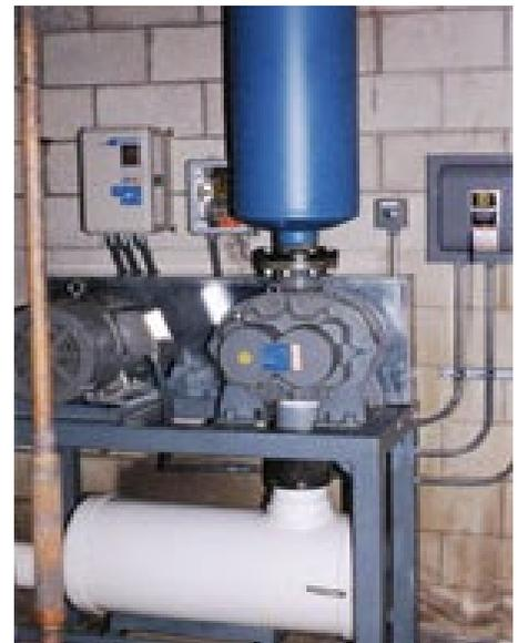
Milk Vacuum Pump and VFD.
