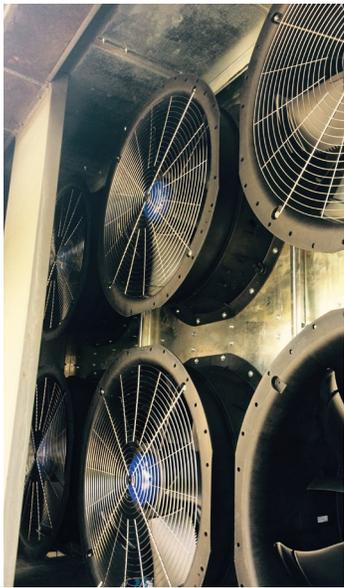
One cell fan wall cooling tower
