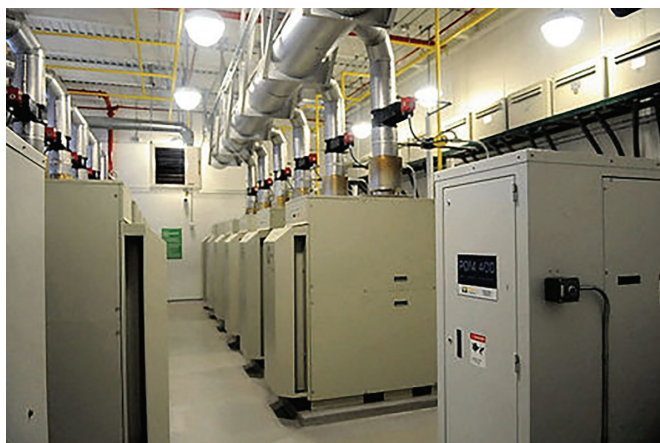
Gas-powered Microturbines at Syracuse University's Green Data Center generate electrical power and heat for hot water and cooling.
