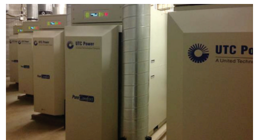
East Irondequiot CSD's CCHP 65kW Microturbines
