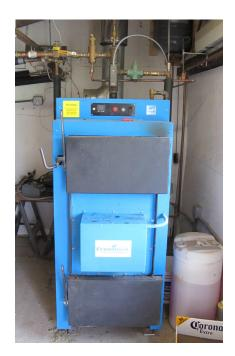
The homeowners wanted to use wood harvested from forest stand improvement activities, eliminate boiler operation from spring through fall, and minimize combustion generated air emissions. Integrating the Econoburn cordwood, two-stage gasification boiler with thermal storage and a solar-thermal system maximized efficiency and reduced emissions.
