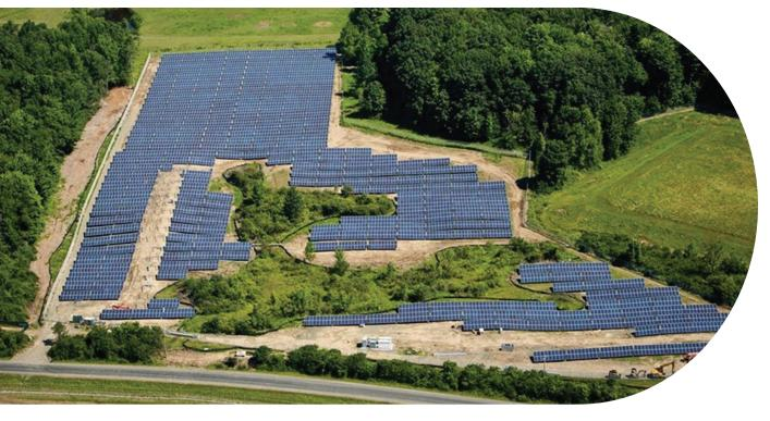
Cornell's Snyder Road Solar Farm in Tompkins County, NY consists of a 2-MW array of solar panels that stretches across 11 acres of Cornell property. The site is part of Cornell's Radiation Disposal Facility. Remediation activities occurred on the site prior to constructing the solar array. (Source: NYSERDA)
