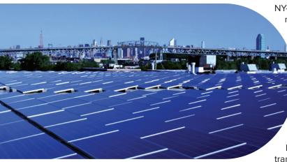
This 408-kilowatt (kW) roof-mounted solar electric system is expected to generate close to 500,000 kWh of electricity a year for Big Geyser, a major nonalcoholic beverage distributor in Queens, NY. Using close to 1,400 solar panels, the solar electric system will generate enough energy to meet the distribution center's annual electric demand. (Source: EmPower Solar)
