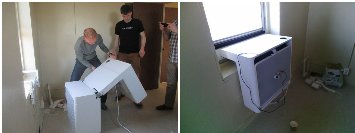
Figure 7. Gradient Unit: Installation Images
