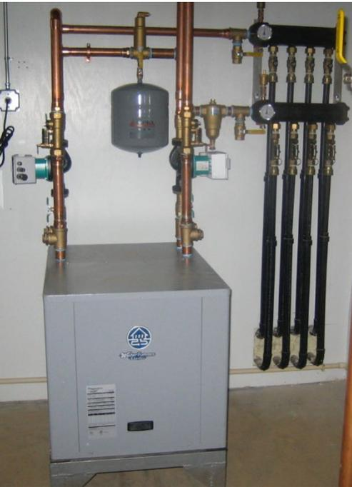
geothermal water-to-water heat pump
