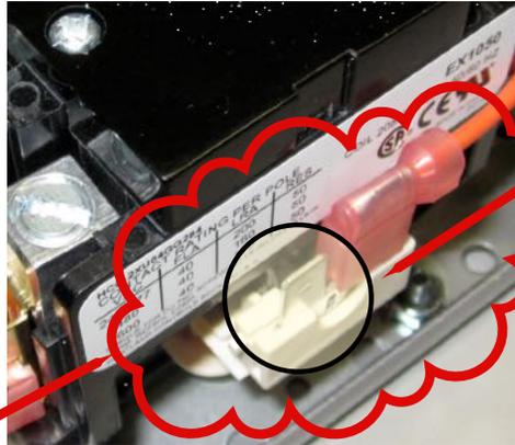
extra terminal on coil circuit of contactor
