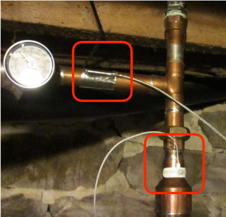
non-insulated surfaced mounted temperature sensors
