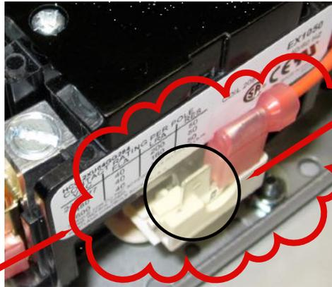
extra terminal on coil circuit of contactor
