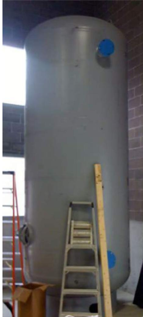
4000 gallon thermal storage tank (before insulation)
