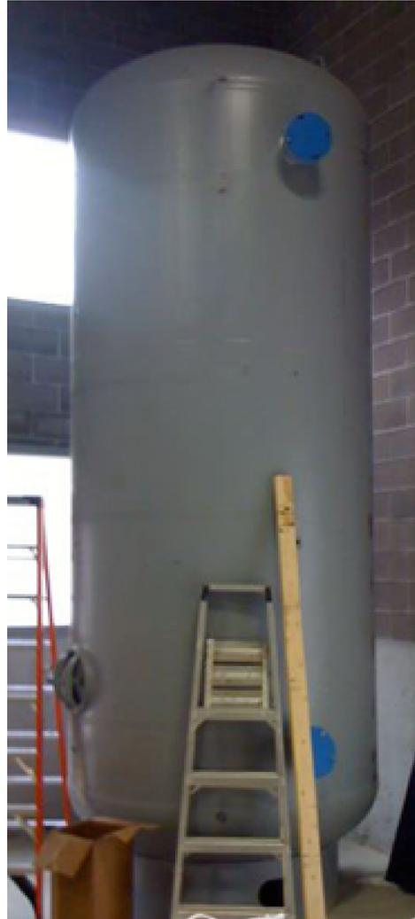
4000 gallon thermal storage tank (before insulation)
