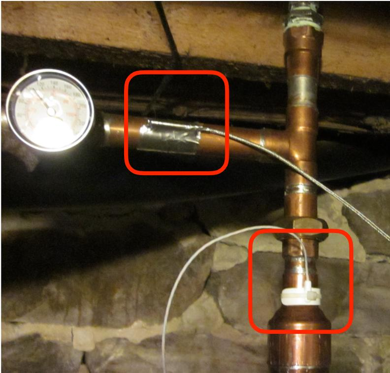
non-insulated surfaced mounted temperature sensors
