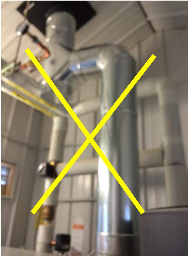
Pellet boiler stack - galvanized pipe - no draft regulator
