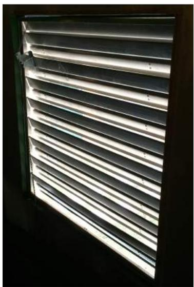
**If motorized louvers are used they must be verified prior to burner operation.**
