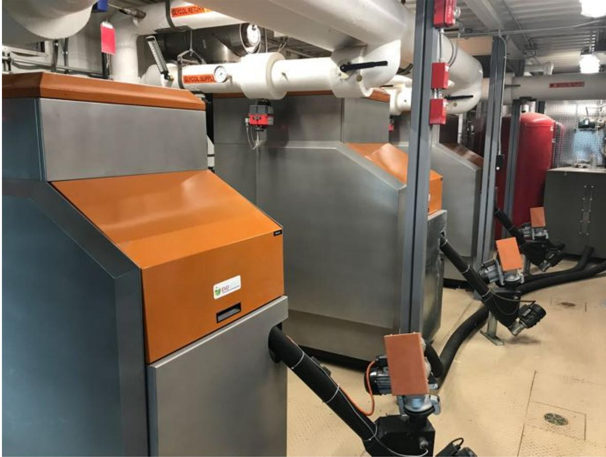
**Boiler firing is based on *measured* total building load**
