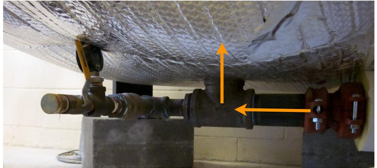
Do not route heat source flow into a vertical top connection (unless tank has inlet flow diffuser)
