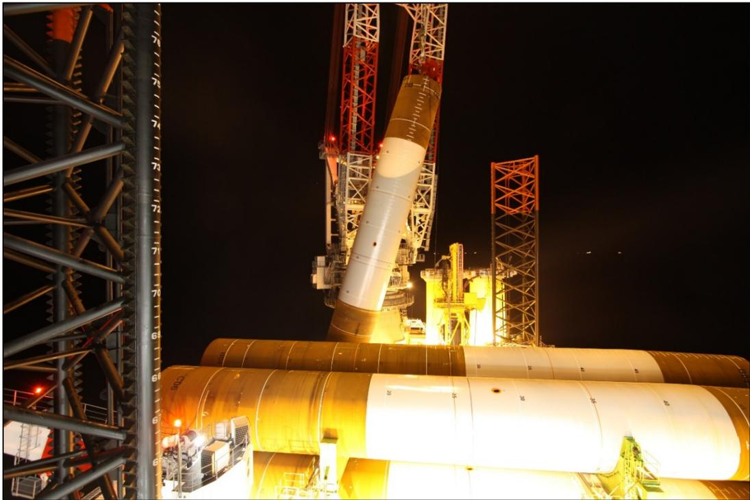
Figure 11.2 Installation of a Transition Piece (Westermost Rough, 2014)
