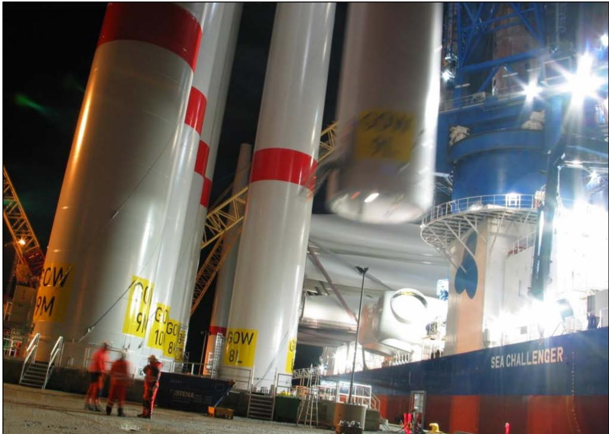
Once positioned at the offshore site, the installation vessel jacks up and connects with a pre-installed foundation via gangway. Installation for each WTG is performed in five lifts; tower, nacelle, and three blades. This method of installing full towers and single blades from a dedicated installation vessel has proven to be an efficient and safe way to install WTGs offshore (Figure 11.9).
