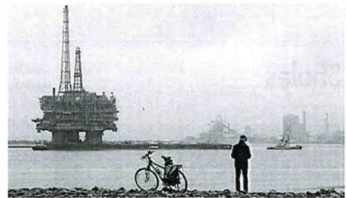
The Brent Delta platform was transported to the Able UK Seaton Port yard in Hartlepool, UK, where at least 97% of the material will be recycled.
