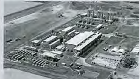
At the QGC Project, Australia, the central water treatment plant recycles salty underground water extracted during gas production.
