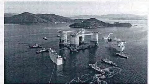
The Appomattox project hull is prepared for its journey from Geogje, South Korea to Ingleside, Texas, USA, to complete the semi-submersible host platform's construction.
