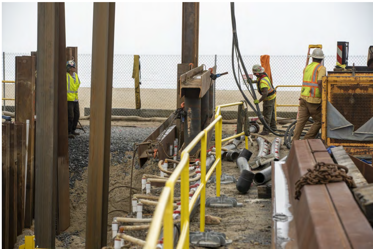
Workers install steel shoring where submarine cables come onshore for the Vineyard Wind project in Barnstable, Massachusetts.
