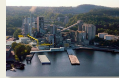
Data Centers / Enabling Infrastructure
