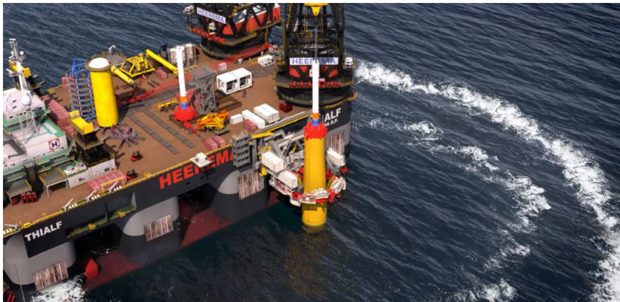
Figure 6.22: Double Big Bubble Curtain Operating Around Monopile Installation
