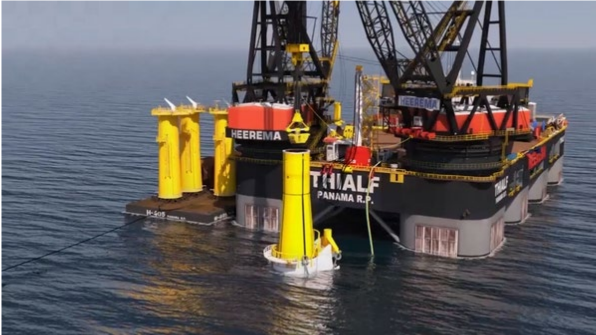
Figure 6.21: Thialf Installing a Transition Piece on Top of a Monopile
