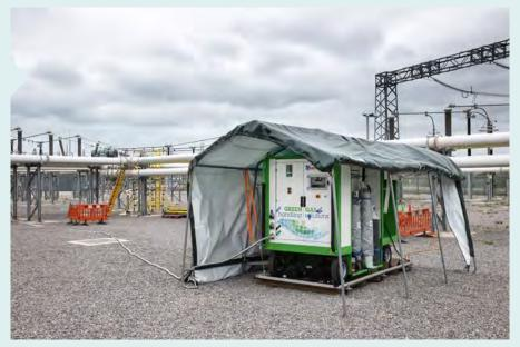
Onsite gas cart used to retro fill existing gas-insulated, high-voltage switchgear, with an alternative low global warming g<sup>3</sup> gas, designed for high-voltage transmission equipment, Richborough Substation, Kent, UK
