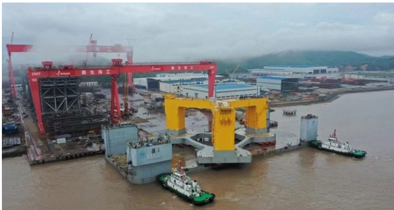
Figure 14. Foundation Assembly and Load-Out at a Port
